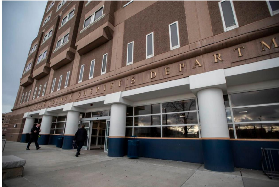
Suffolk County House of Correction. (Jesse Costa/WBUR)
